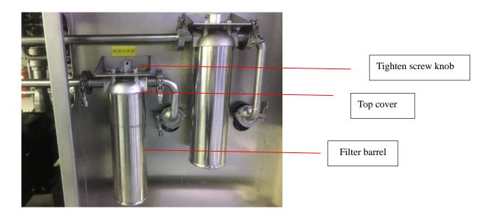
Picture 1 filter barrel
